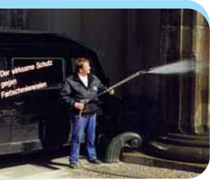
A surface treated with PSS 20 is protected against graffiti and environmental pollution. These can be removed, together with the PSS 20 protective film, simply using warm water. Another great advantage is that PSS 20 forms a transparent film, undetectable to the eye.
